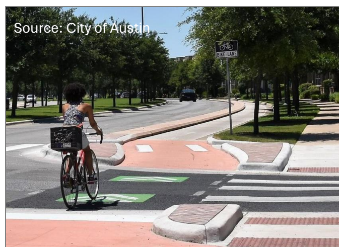
Figure 25. A separated bike lane in Austin with concrete barriers to protect bicyclists from traffic.
